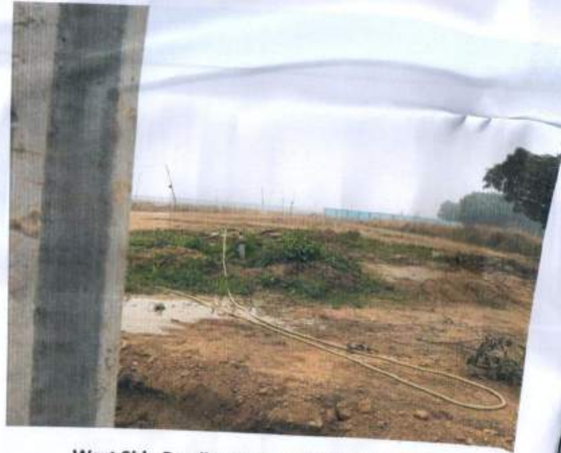
West Side Pending Boundary Wall 115.5 Mtr
